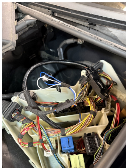
Example of the adapter harness and MAP sensor positioned in the ECU/electronics box during installation.
